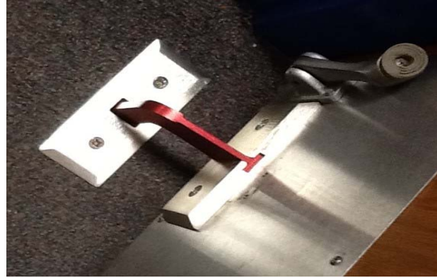
DOOR LOCKS INSTALLED AT HARRISON SCHOOLS
